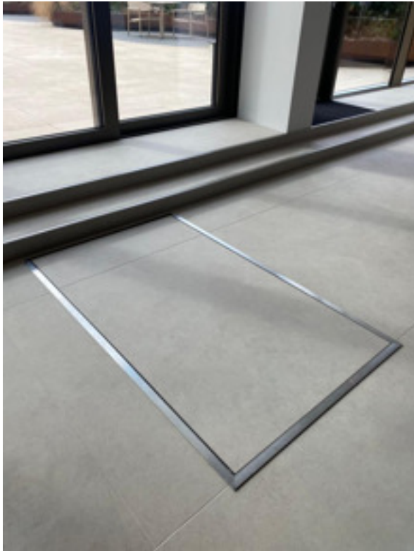
Invisible Step lift concealed in the floor of a prestigious London office building.
