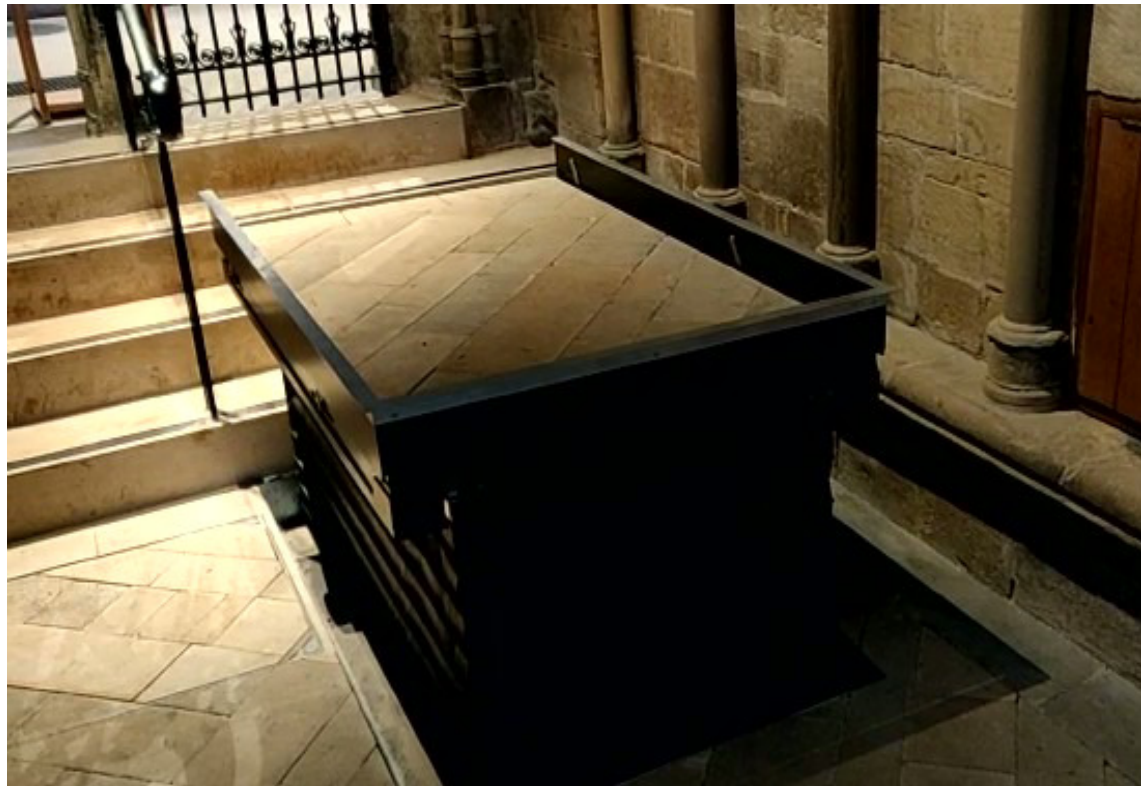
Invisible Step Lift raised and in use providing wheelchair access inside a Heritage Grade 1 listed Cathedral in England.
