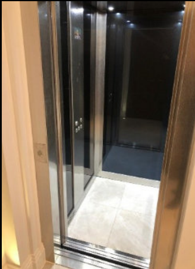
Hydraulic Passenger Lift in a Mansion
