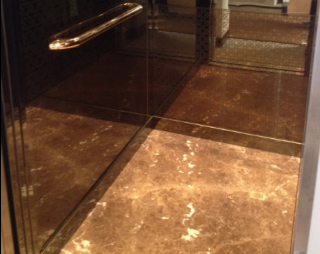
Close up picture of the lift cabin floor.
