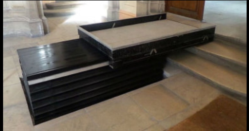
Lift in use (having risen vertically then extended horizontally)
