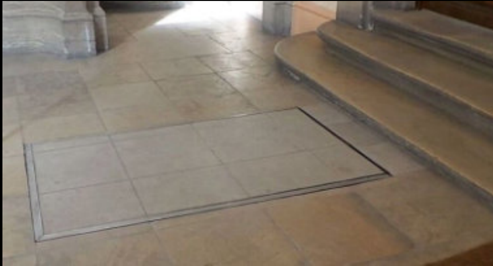
Lift in the rest position concealed under the floor
